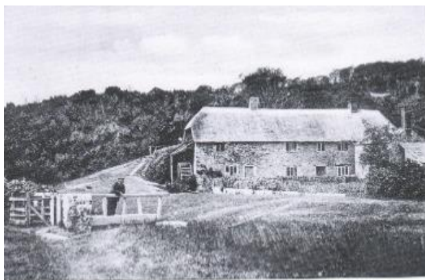
The Old Mill in 1900, one of nine mills on the River Lym between its source near Hunters Lodge and the sea at Lyme Regis. It is the last building in the parish, the bridge in the foreground being part of the Dorset/Dorset boundary.
